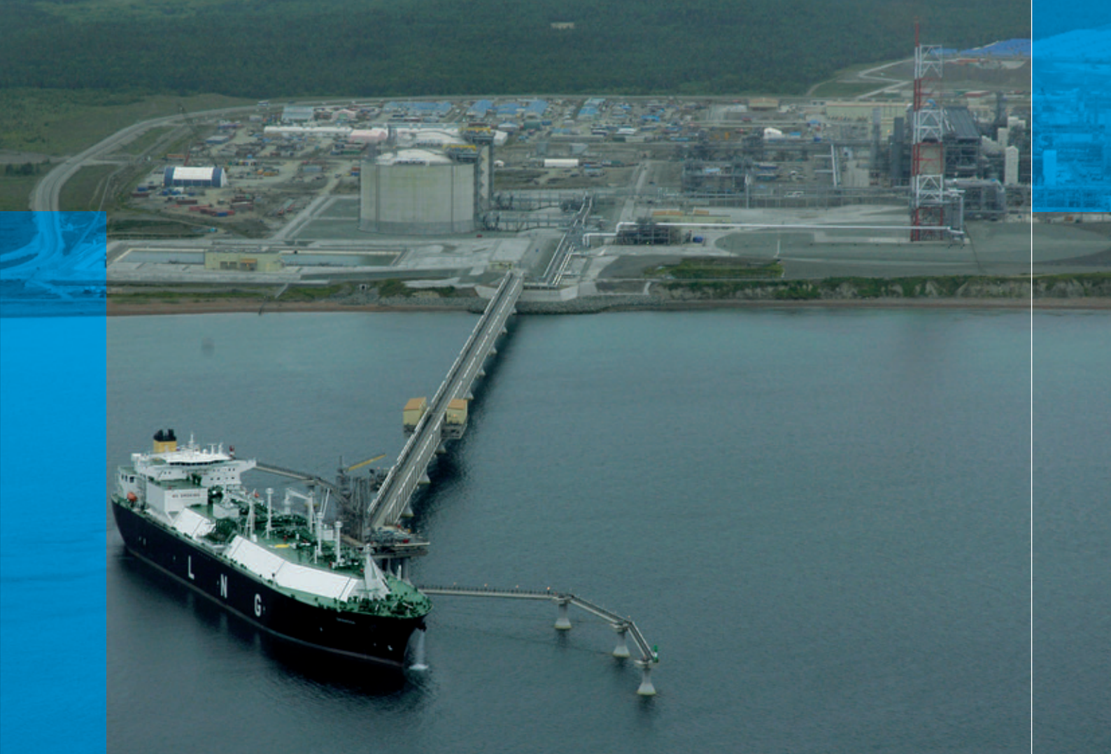
Figure 1. Sakhalin II LNG Plant with Shell DMR Process (Courtesy of Sakhalin Energy)
